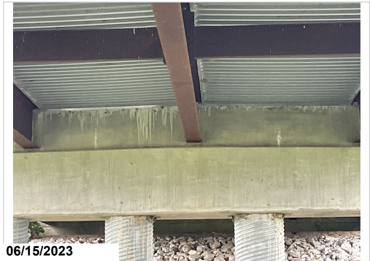
concrete above caps at bents have a few vertical cracks with light efflorescence.
