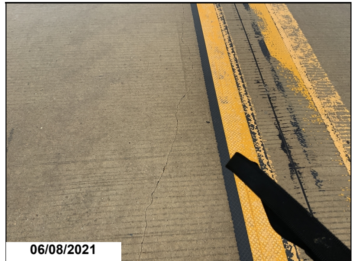
Typical longitudinal crack in approach slab.
