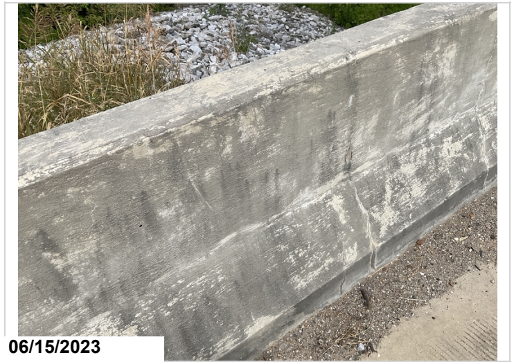
Bridge rails have vertical cracks spaced every 4' some with light efflorescence.
