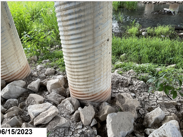
Typical rust on cmp around steel piles
