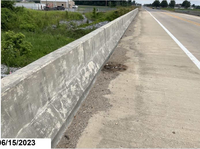
Typical debris in gutters
