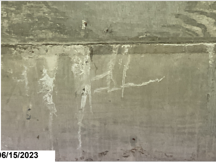
Typical abutment crack
