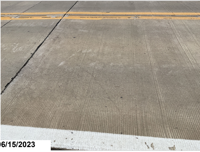
All approach slabs and gutters have hairline and cs2 cracks.
