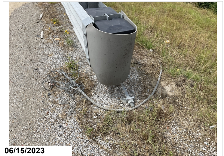
Abutment #2 left approach rail cable broken.
