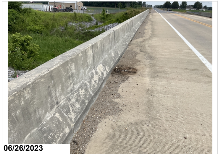
Typical debris in gutters
