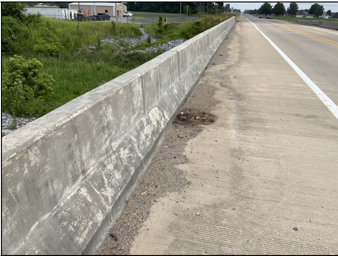
Typical debris in gutters
